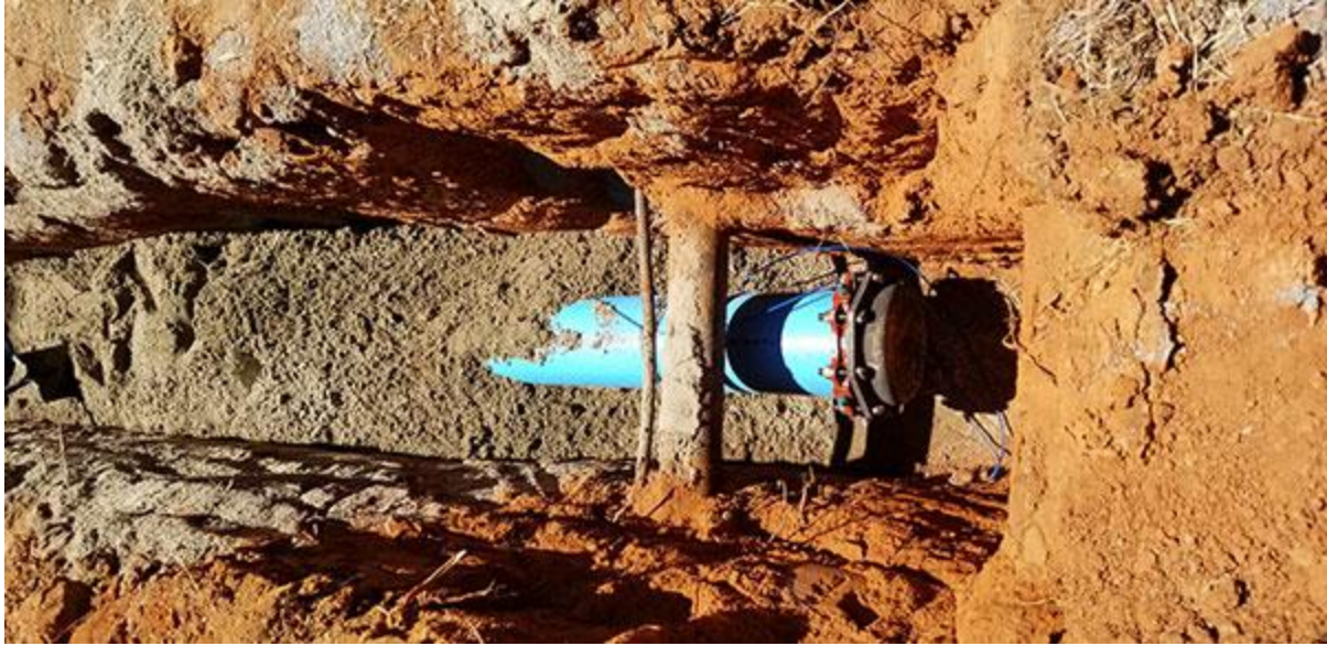
Figure I-4 Foresthill Road Pipeline
