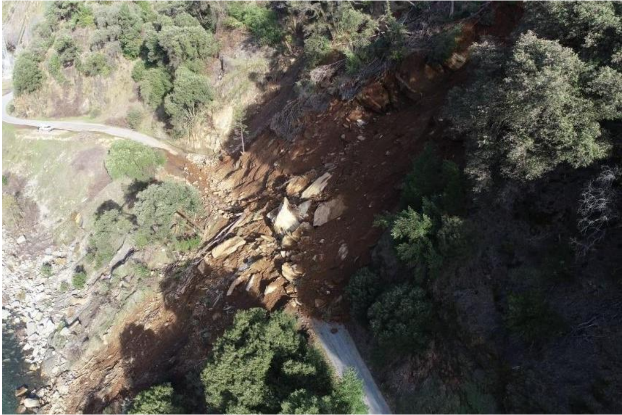
Figure 4-89 2018 Interbay Road Landslide
