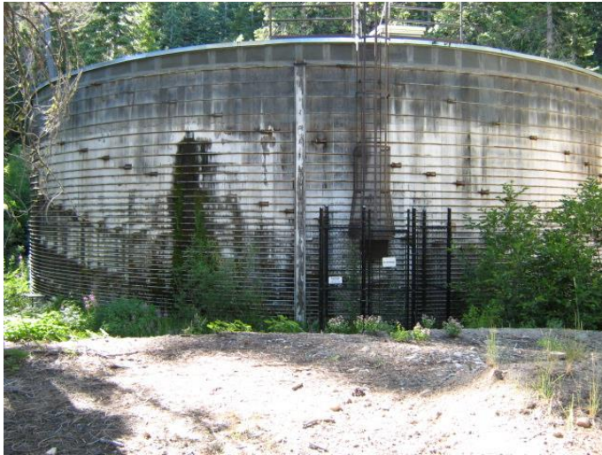
Source: Tahoe City Public Utility District
