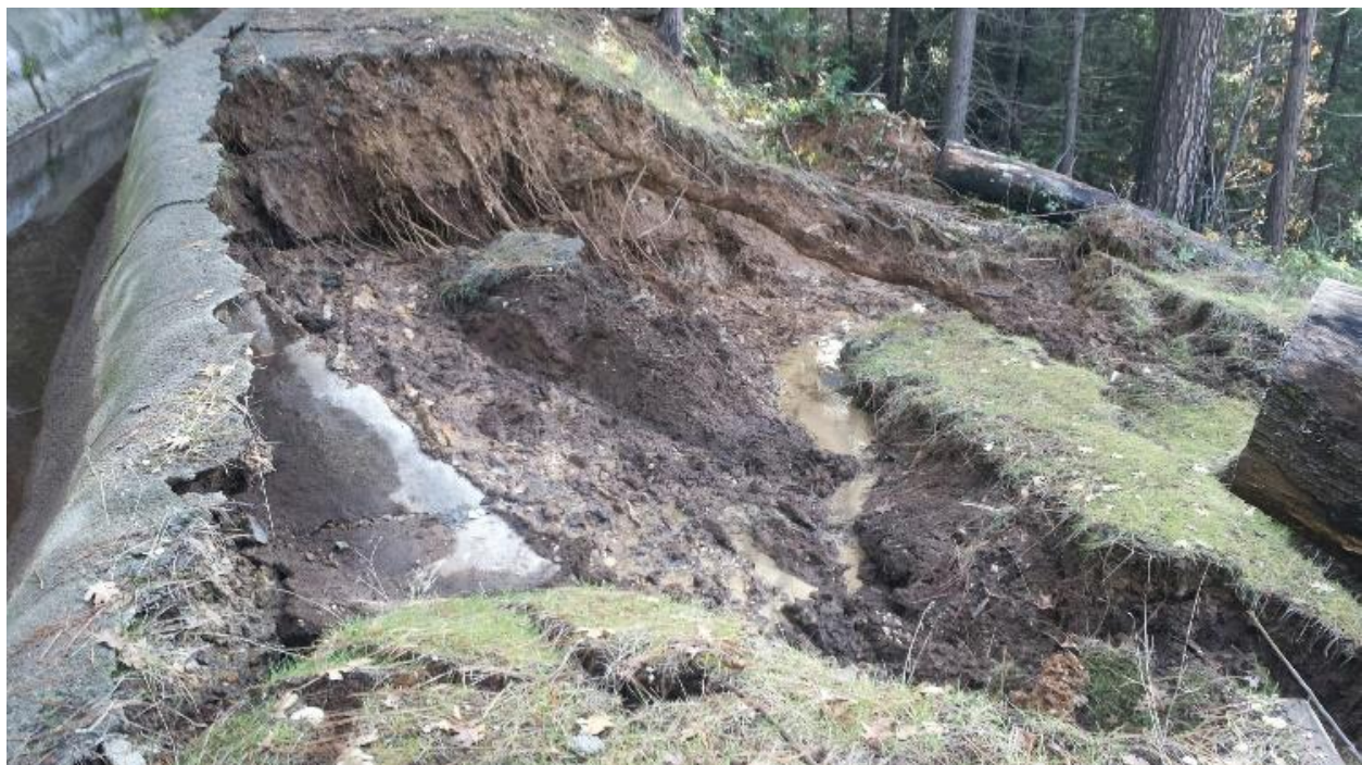
Figure R-11 Pulp Mill Canal 2017
