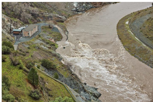
Figure R-5 American River Pump Station
