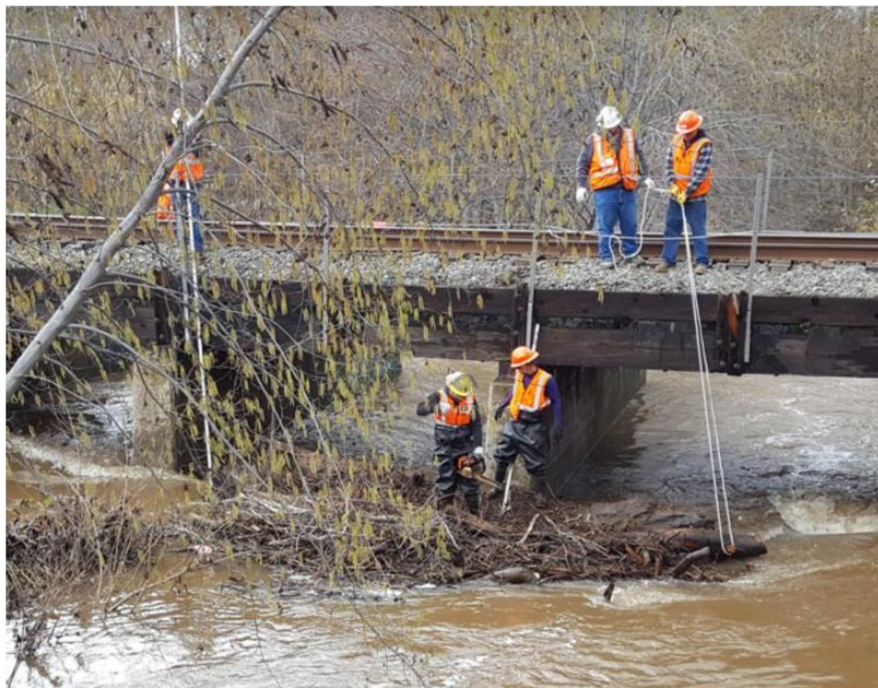
Figure C-7 City of Lincoln – Flooding at Railroad Bridge on January 17, 2019
