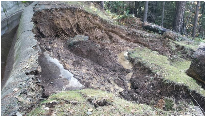
Figure R-7 Pulp Mill Canal 2017
