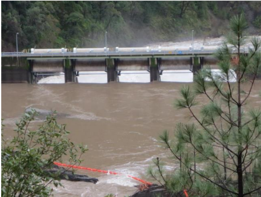
Figure R-6 Afterbay Dam
